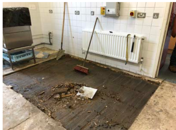
The work to the floor was extensive, and messy!
